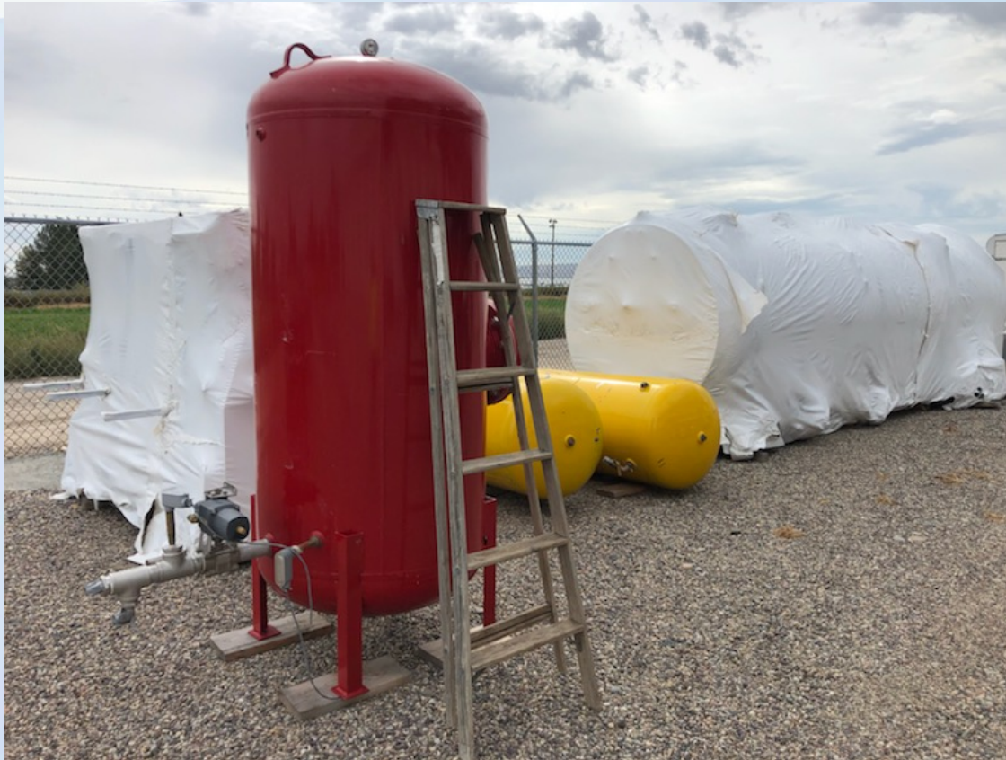
Fire Suppression Deluge System Water Tank
